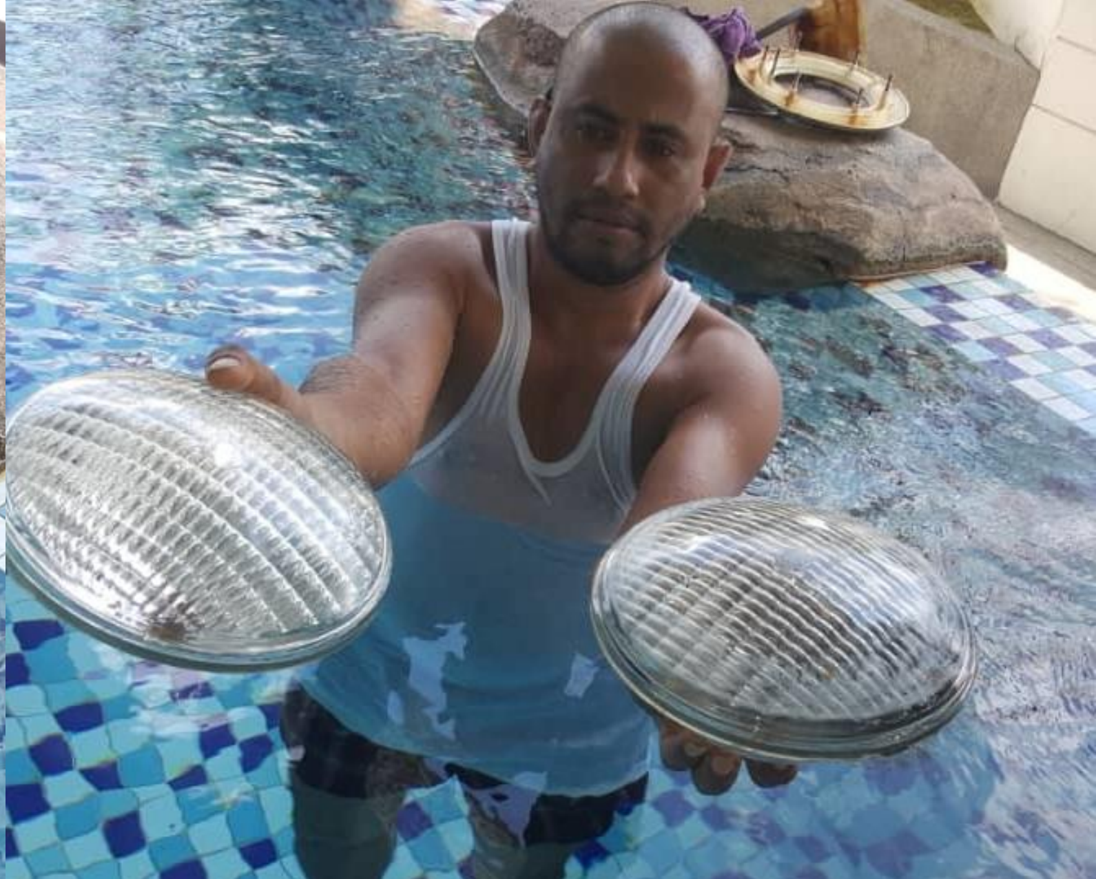
Replacement of underwater light
