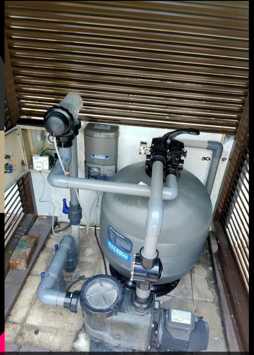
Fixing new salt machine, filter & light
